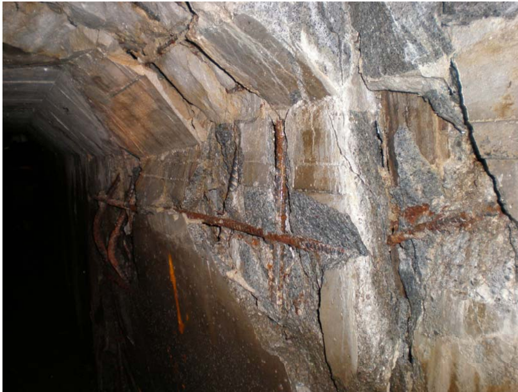
Above: High up in the Southern Alps, the 100 year old 'Old Big Wainihinihi Tunnel' in state of failure due to earth movement
