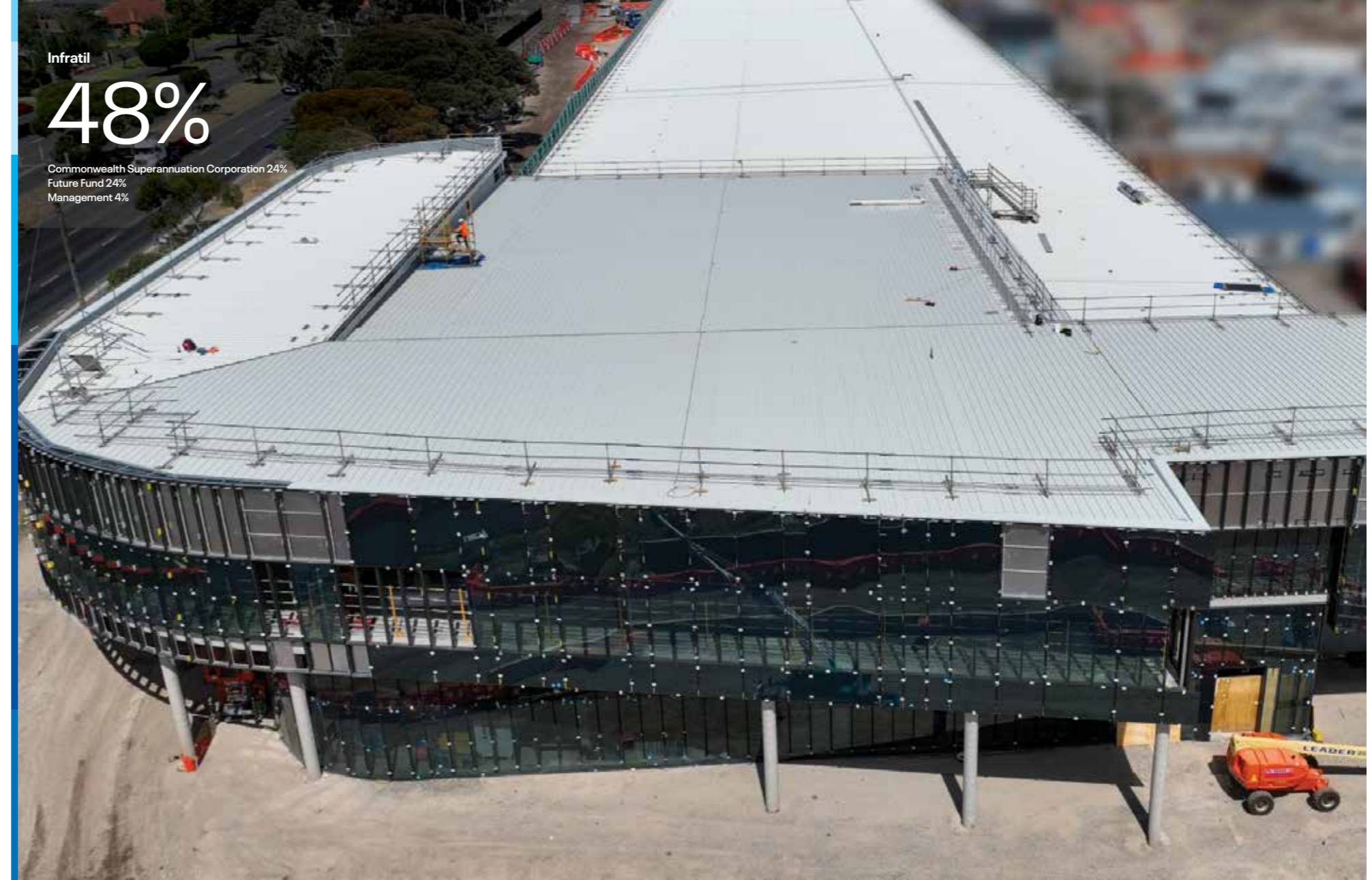
Brooklyn 1 under construction in Melbourne
