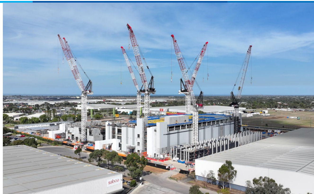
Construction at CDC's Laverton campus, Melbourne.
