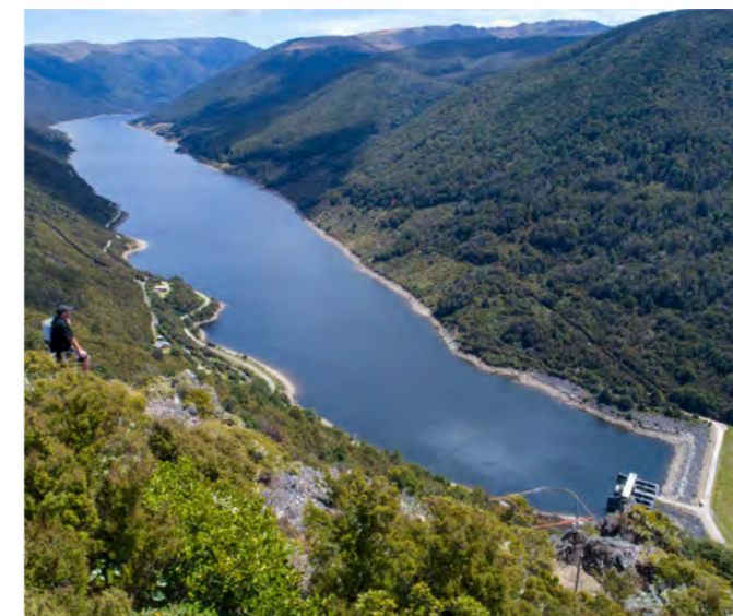
Manawa Energy's Cobb River Hydro-electric Power Station, New Zealand
