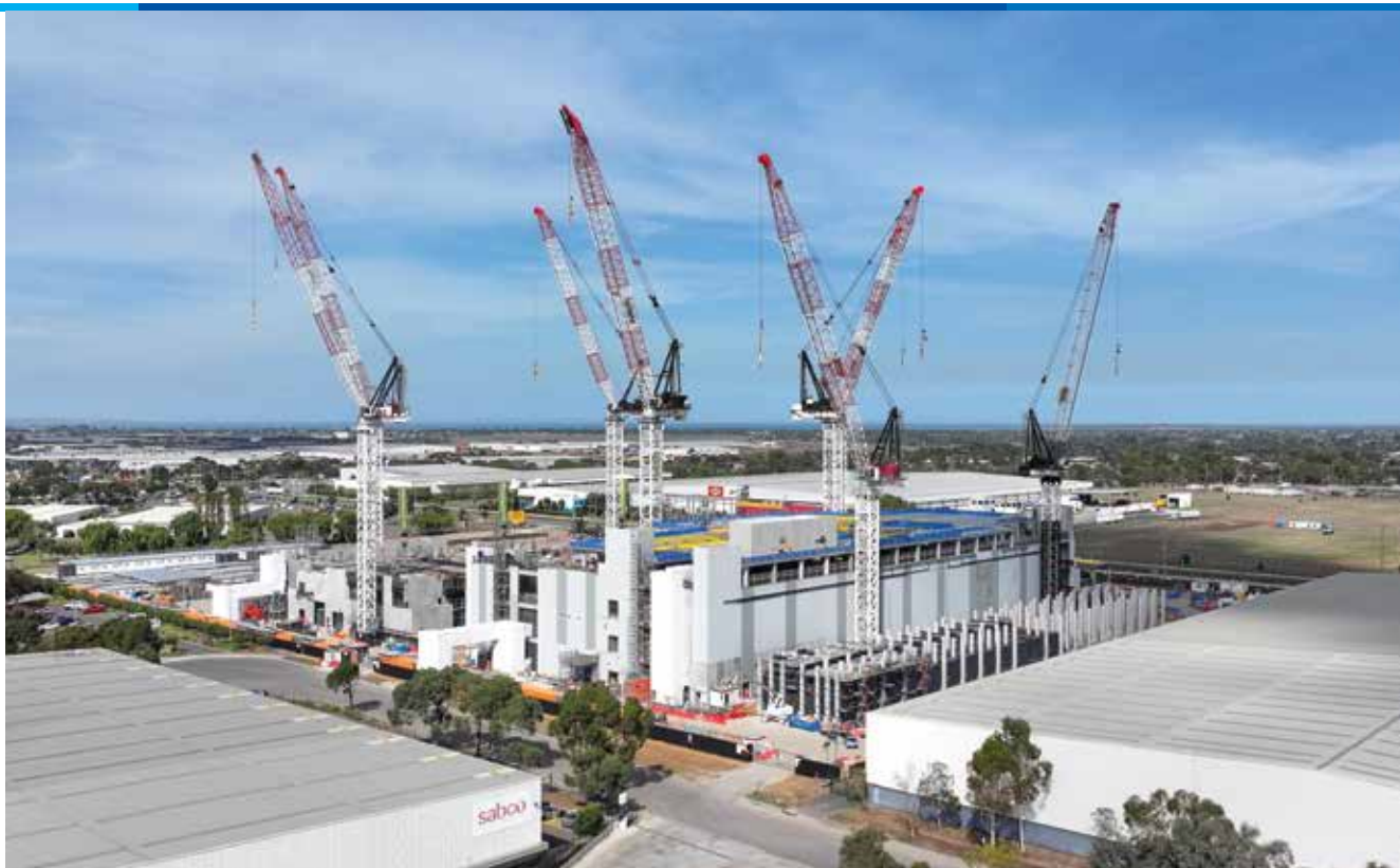
Construction at CDC's Laverton campus, Melbourne.
