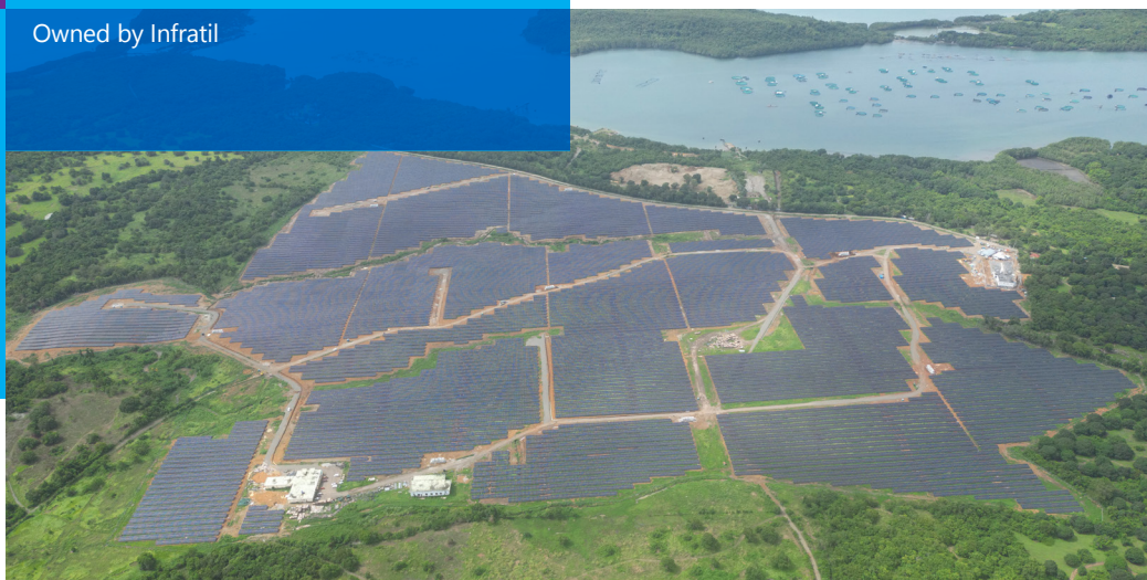
Gurin's 75MW solar power plant in Zambales Province, Philippines
