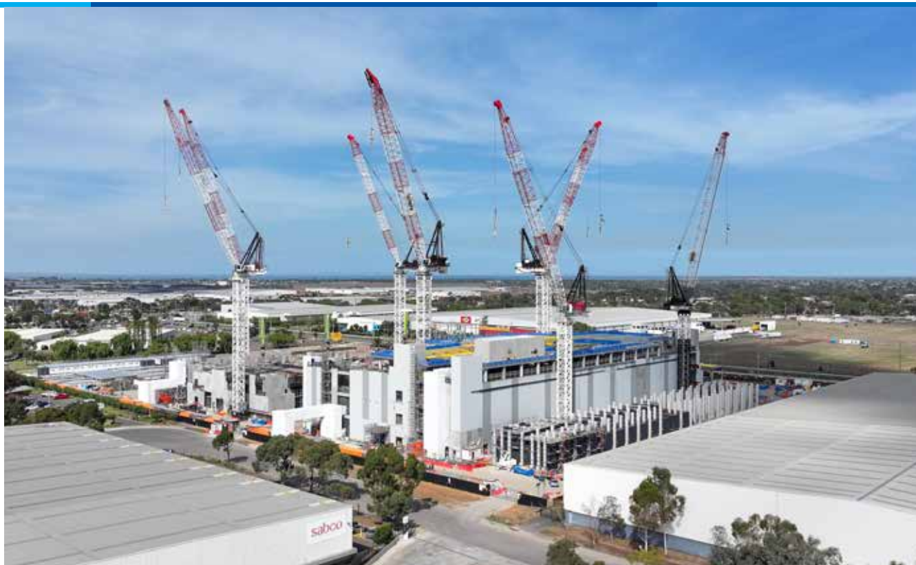
Construction at CDC's Laverton campus, Melbourne.
