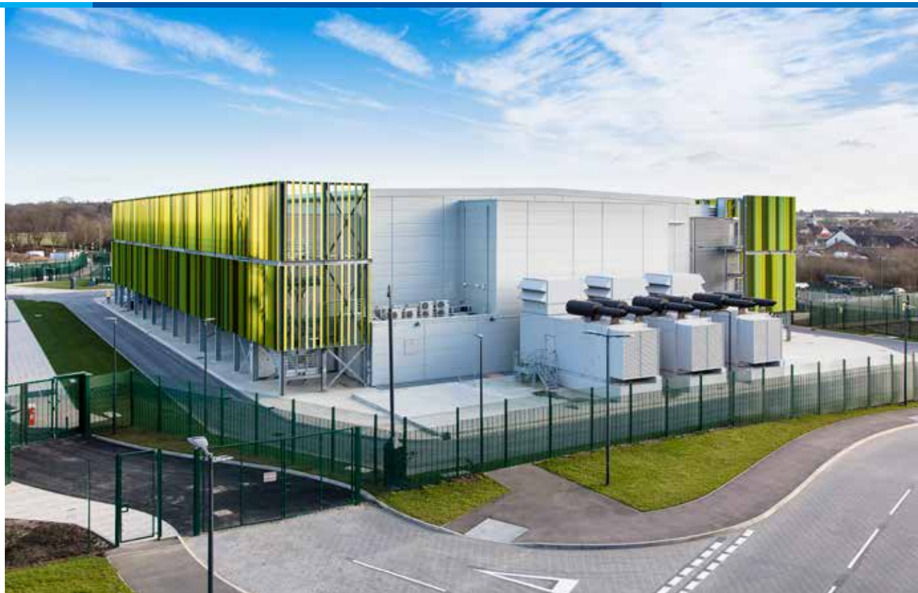
Kao Data's Harlow Campus, located between London and Cambridge, United Kingdom.
