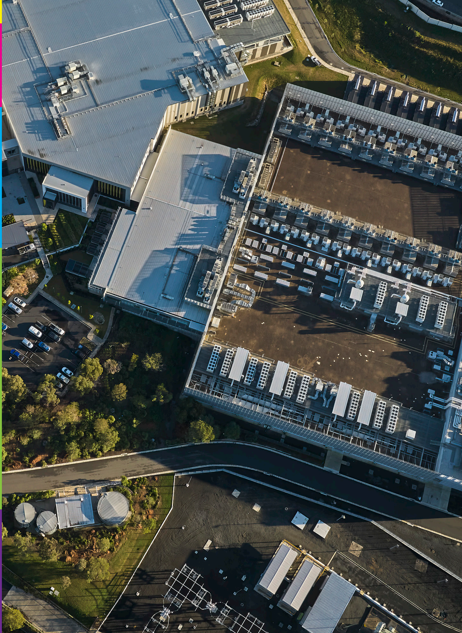
Eastern Creek data centre
