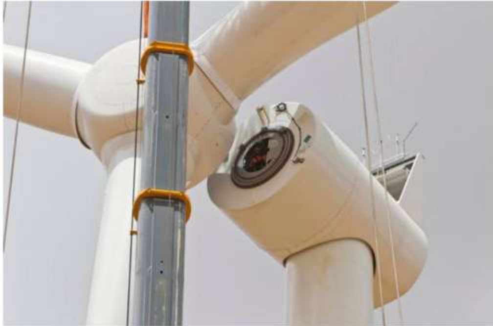
Connecting turbine blades to a tower.
