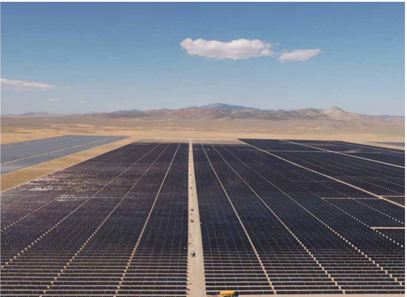
Qscan magnetic resonance imaging machine. Vodafone 5G installation Auckland. Tilt Renewables' Waipipi wind farm, Taranaki. Longroad Energy's utility scale solar installation Texas
