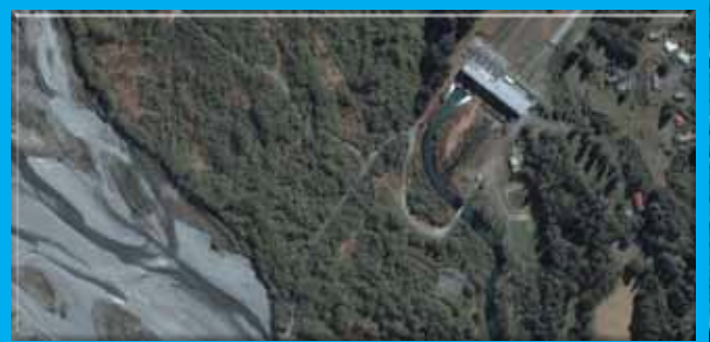
TrustPower's Coleridge Power Station
